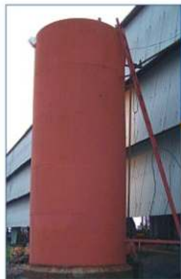
Oil Storage Tank
